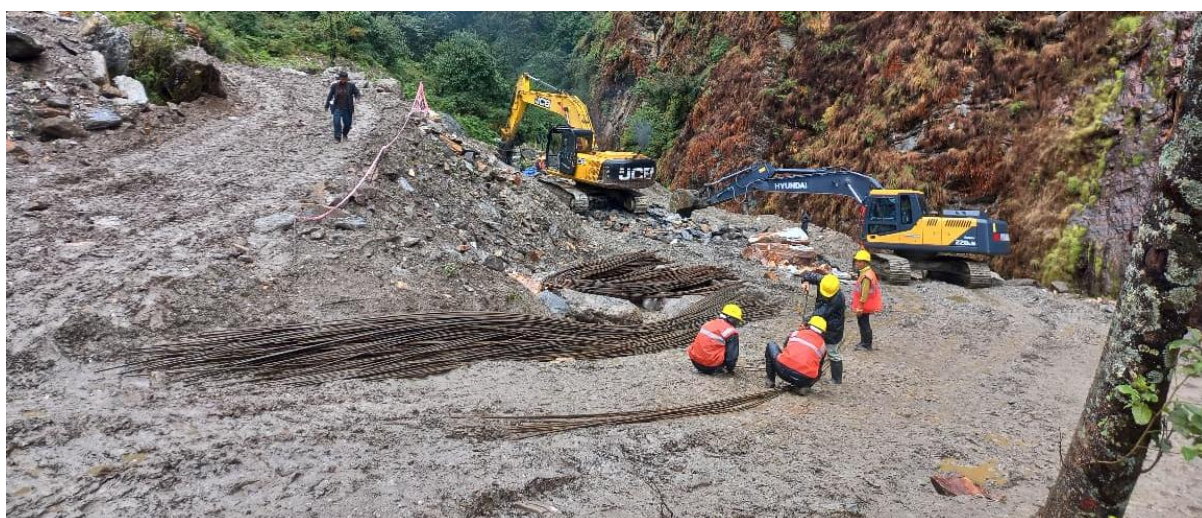
Figure 9: Reinforcement straightening and preparation works being carried out
