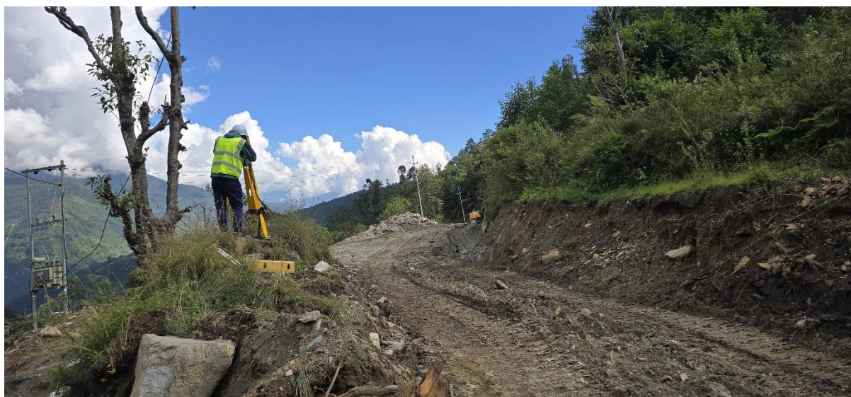
Figure 11: HRP Excavation along with Survey works going on
