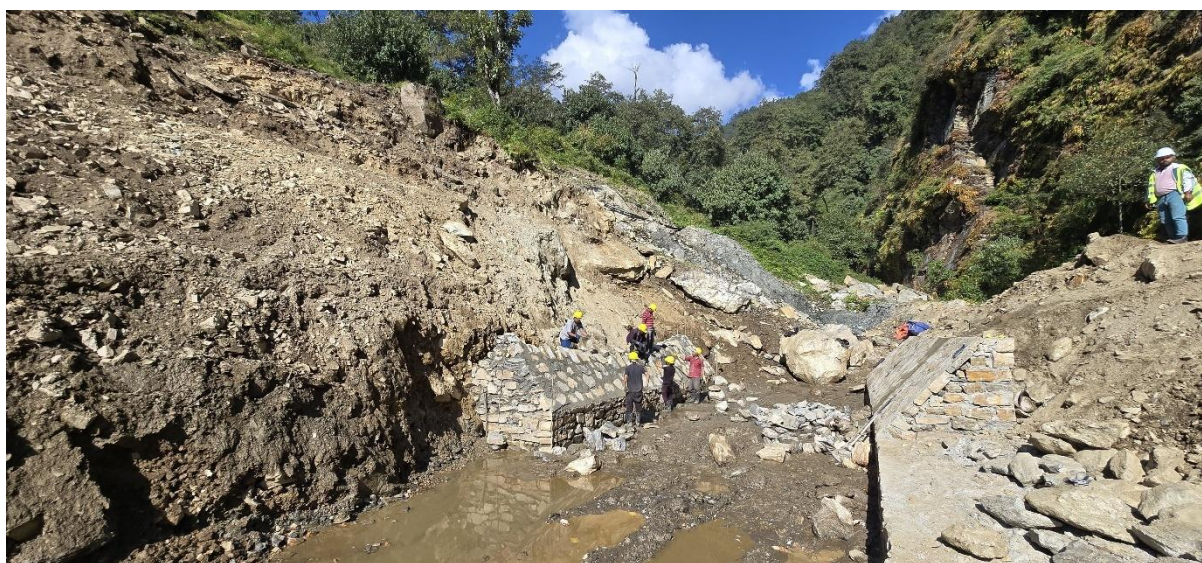
Figure 4: Ongoing works of stone masonry works at settling basin
