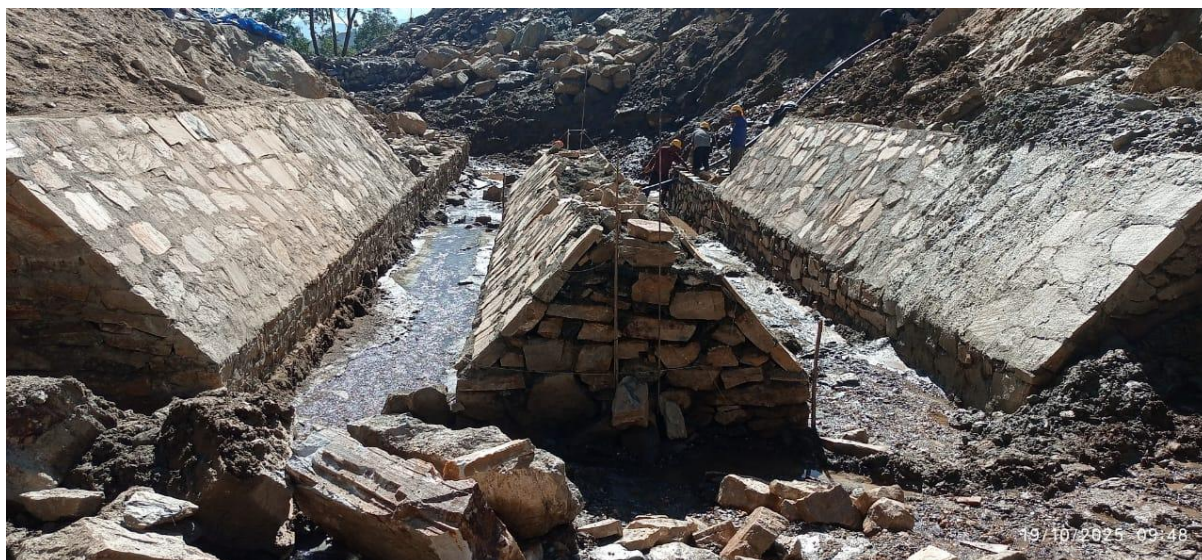
Figure 3: Ongoing works of stone masonry works at settling basin
