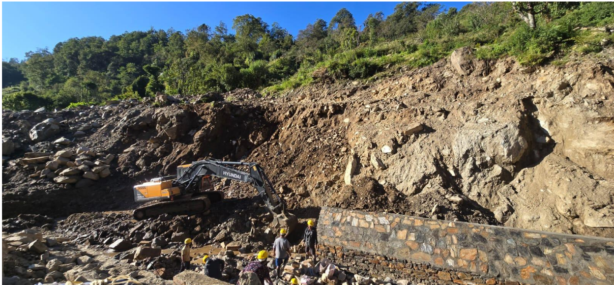
Figure 1: Stone masonry work along with site clearance at settling basin
