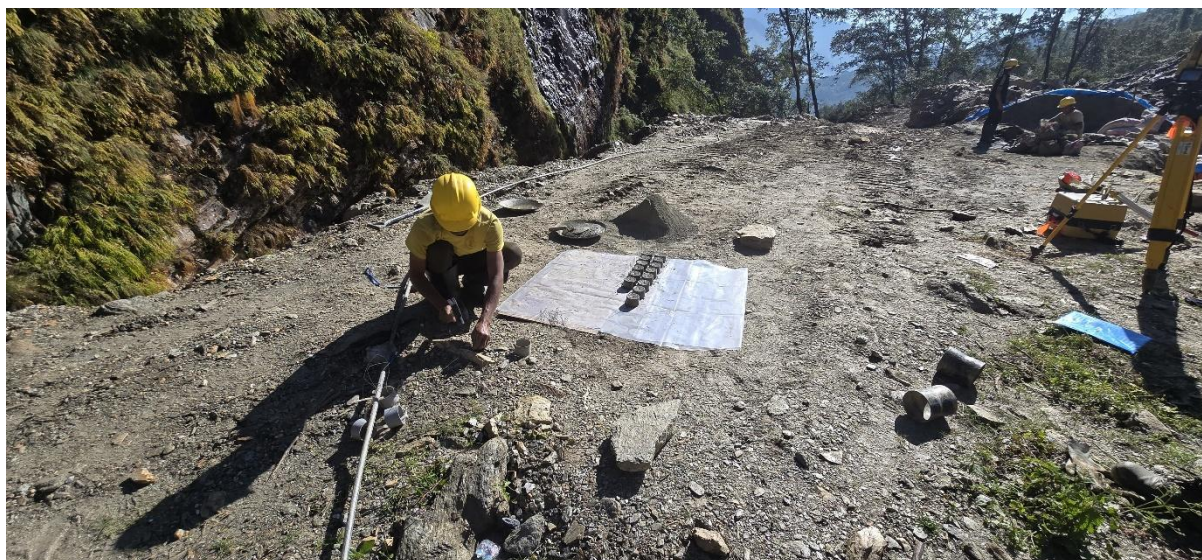
Figure 8: Preparation of clear cover blocks in progress
