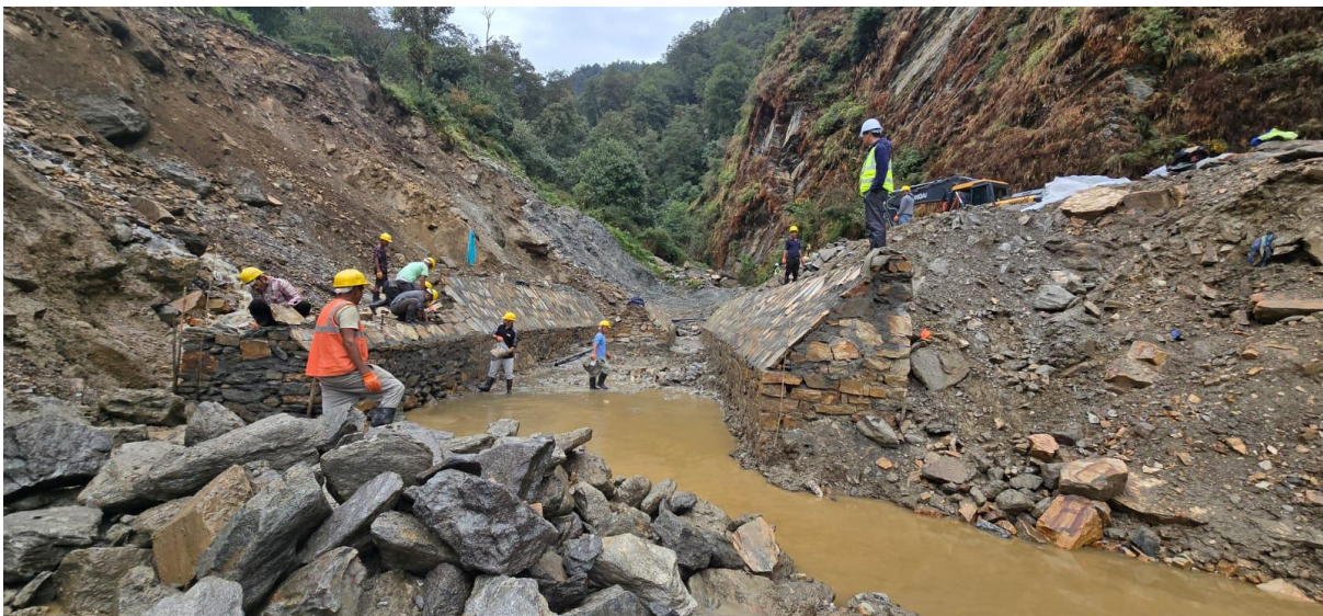
Figure 2: Stone masonry work in progress at the settling basin
